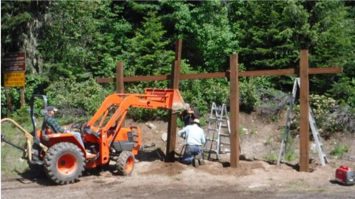
**Canyon Junction sign reconstruction.** Dick Monaghan with his tractor lifts a post for placement. Carl Stone and Geoff Billing guide the post into the hole. The posts are 8x8 inch by 12 feet long w4x6 cross piece that carries the signs.
